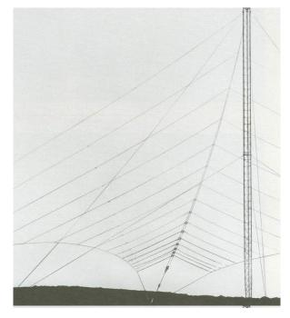
The antennas are easy to erect. The 75ft (22.9m) tower which supports the antenna is supplied in nested sections with a special erection fixture that simplifies installation.
